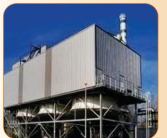
Air Cooled Condensers
